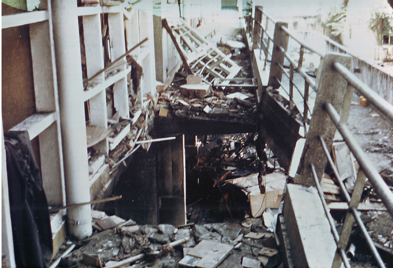
After the explosion at the Brink Bachelor Officers Quarters, Reynolds went back to the building to salvage items. While there she used her camera to take photographs of the after effects of the explosion; the balcony of the room next to hers demolished.
